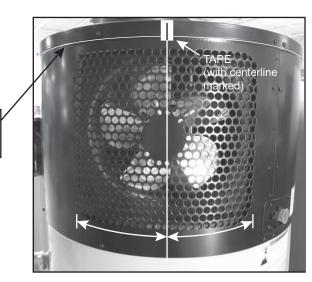
Align the centerline of the template with the "taped" centerline and the top of the template sheet with the lip edge of the jacket top. NOTICE: For proper operation the template must be aligned with the center of the outlet vent. Use your finger tips to locate the outside edges of the vent. outlets. The vent outlets should not be outside the template borders.
