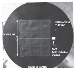
Align the centerline of the template with the "taped" centerline and the top of the template sheet with the center of the two top screws. NOTICE: For proper operation the template must be aligned with the center of the inlet vent.
