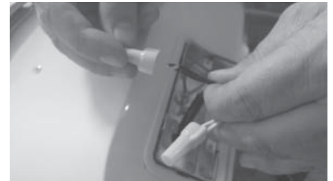
Figure 18 - Connecting the electrical wires.
