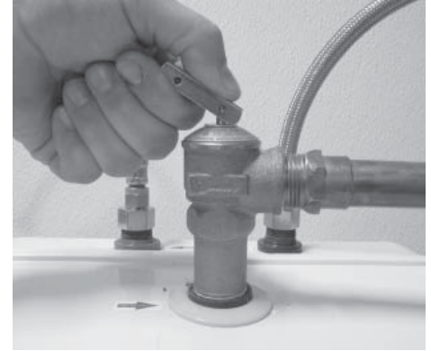
Figure 31 - T&P Relief Valve
